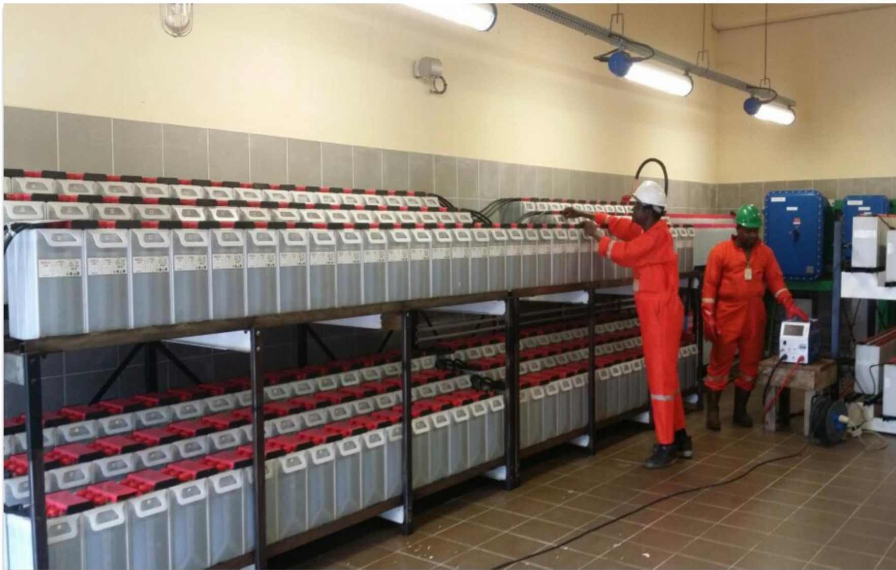
↑ SJV OFFSHORES Personnel at work in a Gas Plant Facility For Batteries Installation/Load Bank Testing
